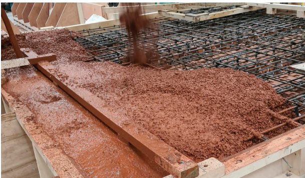
> Concrete is poured
