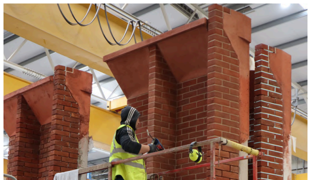
> Pointing is completed
