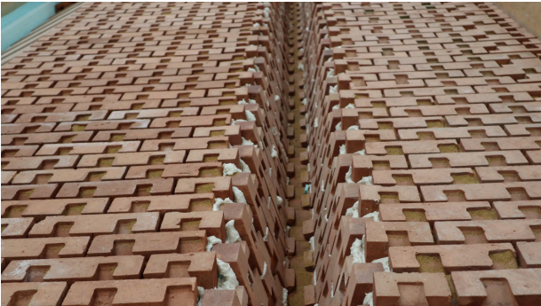
> Brick slips are placed in the mould
