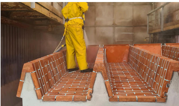
> Panel is sprayed down with water
