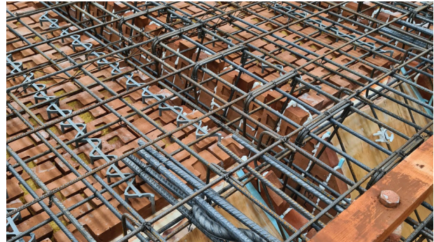
> Steel reinforcement is placed in the mould
