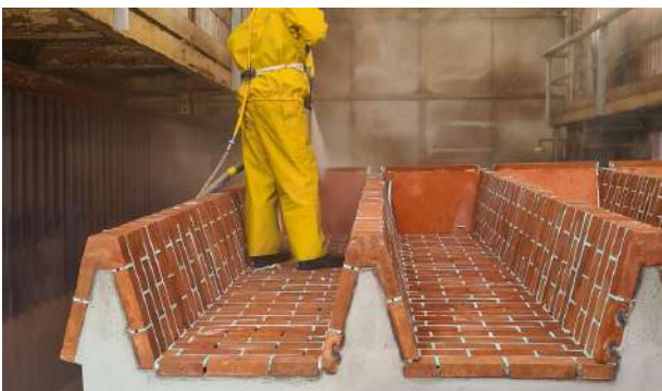
› Panel is sprayed down with water
