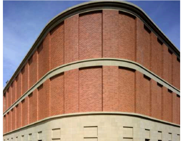
> Bramall Music Building, Birmingham
