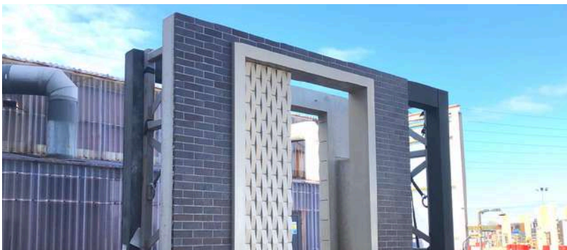
› Osiers Road, London
