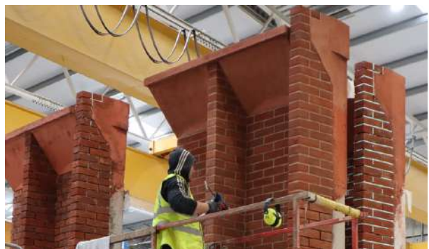
› Pointing is completed
