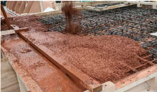
› Concrete is poured
