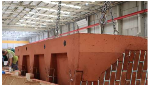
› Panel is lifted out of the mould
