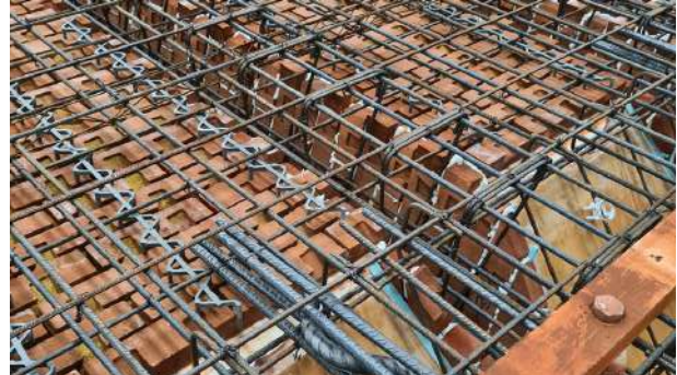
› Steel reinforcement is placed in the mould
