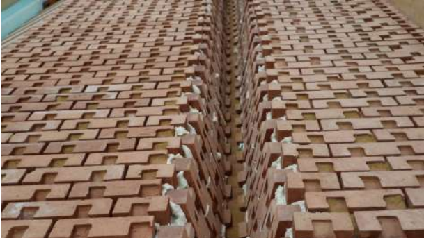
› Brick slips are placed in the mould
