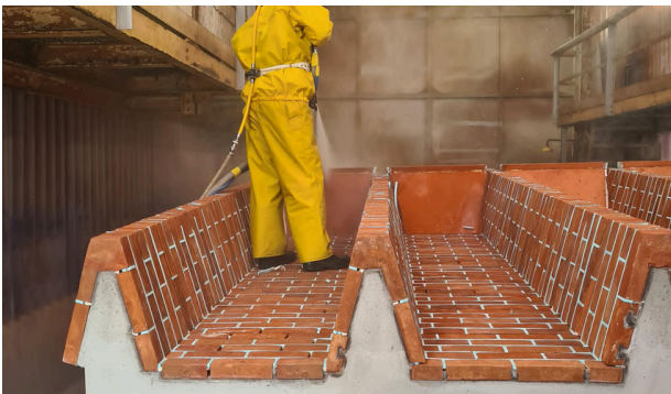
› Panel is sprayed down with water
