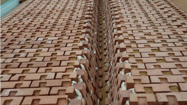
› Brick slips are placed in the mould
