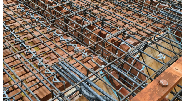
› Steel reinforcement is placed in the mould
