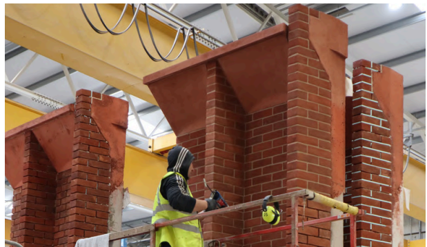
› Pointing is completed
