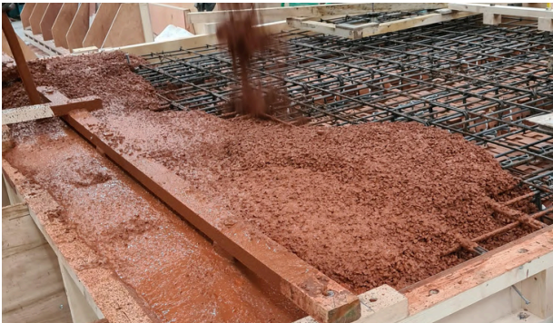
› Concrete is poured
