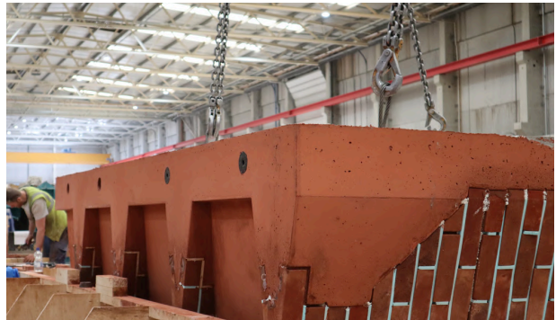
› Panel is lifted out of the mould
