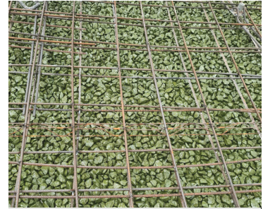
Steel cage is placed in the mould as re-inforcement
