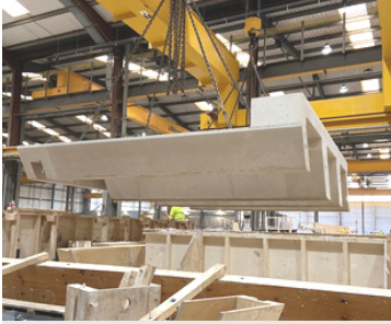
Panel being lifted out of the mould
