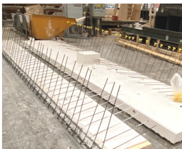
Reinforcement is placed for a two-stage cast
