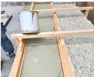
Rubber is poured for the bush-hammered finish
