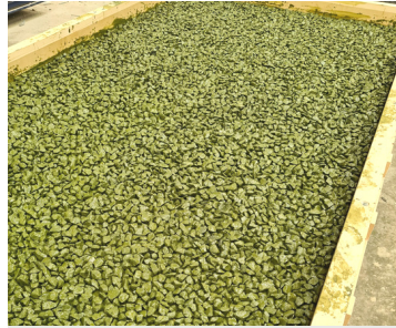
Aggregate is in place
