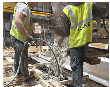
Concrete is poured
