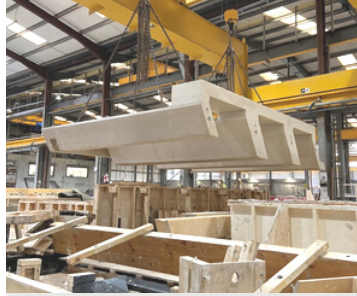
Panel being lifted out of the mould
