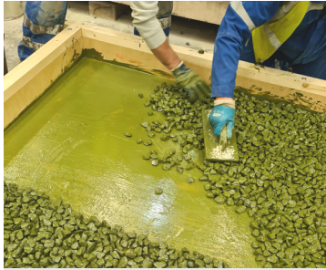
Aggregate is hand-levelled
