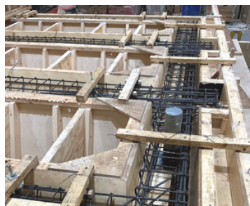
Casting of a unit with re-bar in place
