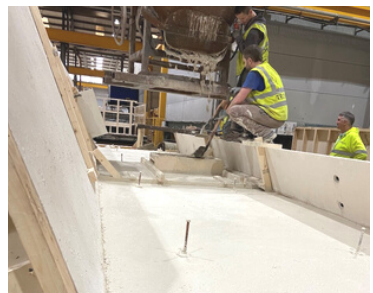
Concrete is poured and trowled by hand
