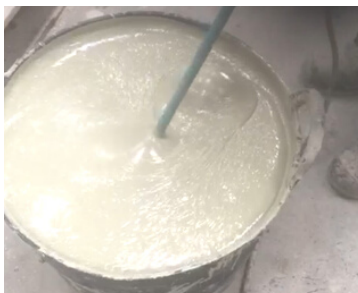
Hand mixing of the rubber
