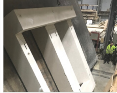
Panel being turned on a steel turning rig
